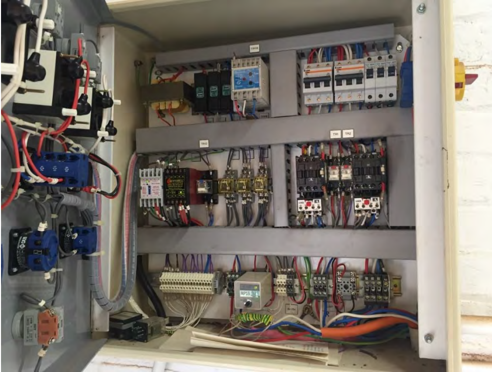
Figure 16-5: Hospital Well SPS MCC panel – this panel is to be replaced
