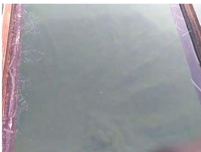
Figure 3-5: Uneven Sludge Blanket with Mounds Visible.
