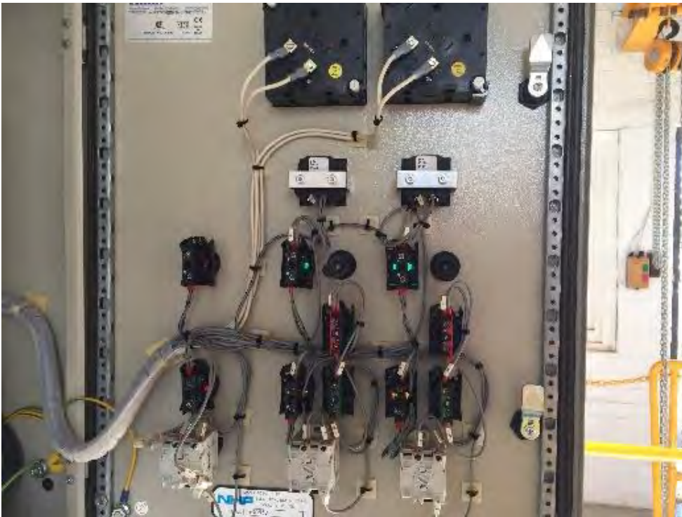
Figure 16-10: Queen St SPS control panel – door wiring
