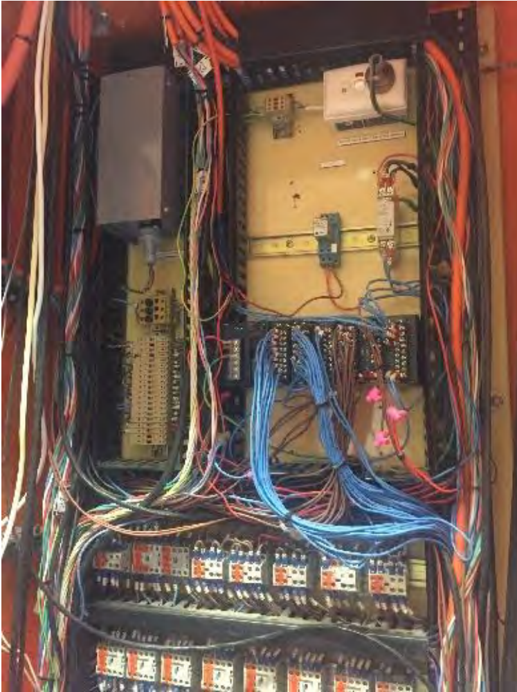
Figure 16-23: WTP control wiring
