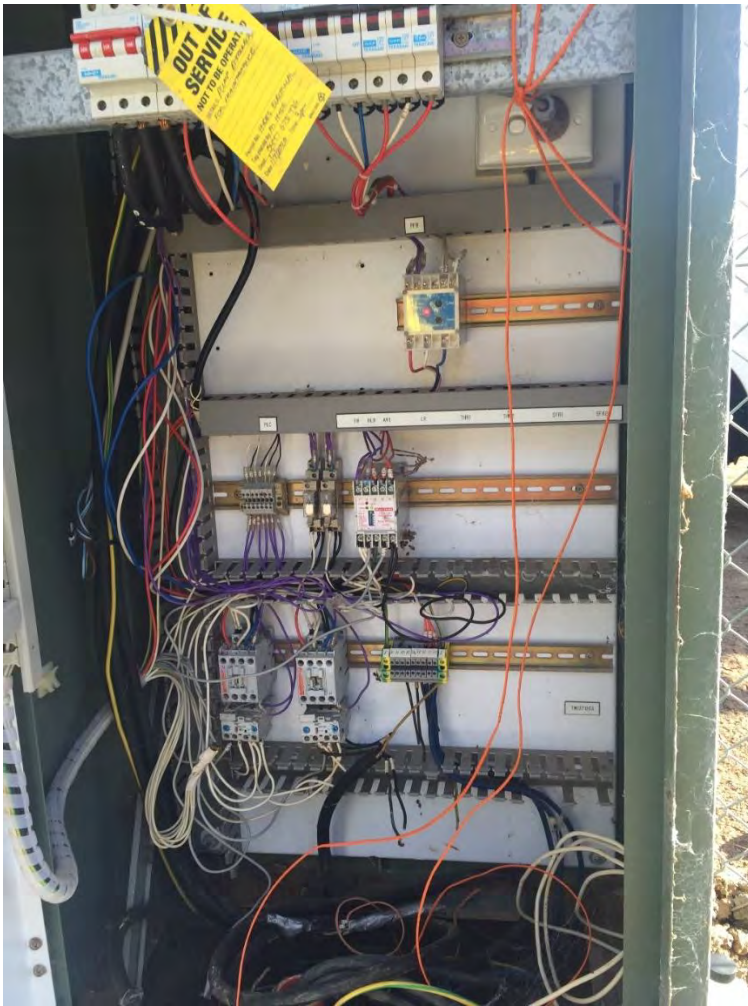
Figure 16-4: East Hay SPS MCC panel – wiring condition poor
