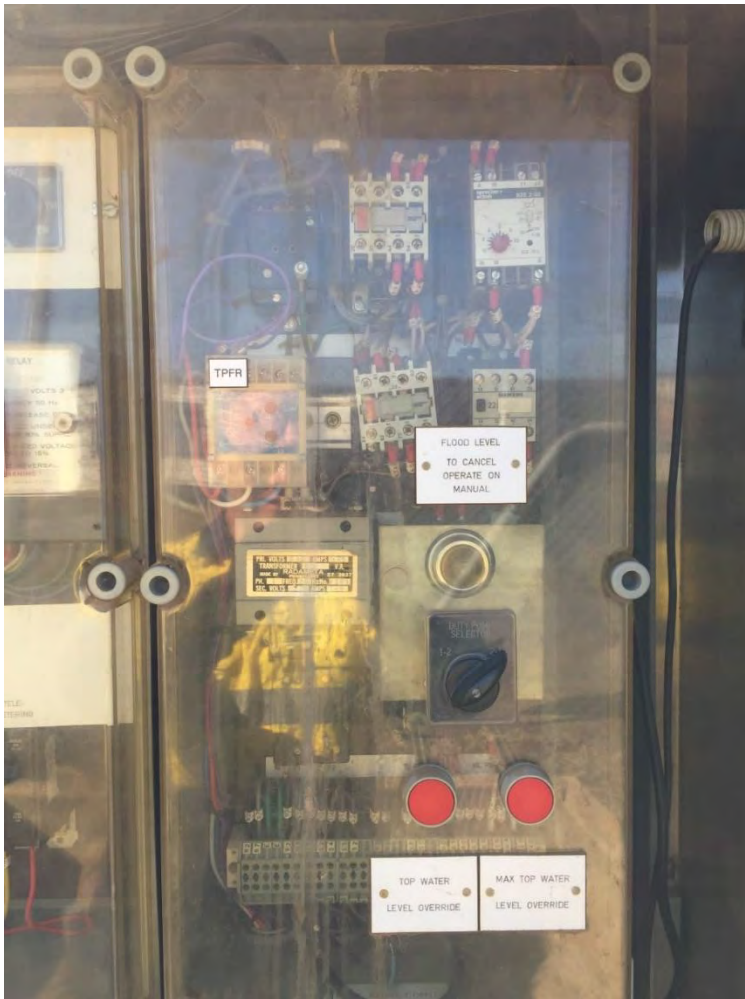
Figure 16-17: Russell St SPS MCC starter / control panel internal
