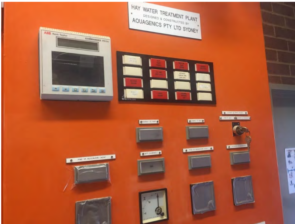
Figure 16-21: WTP MCC control door
