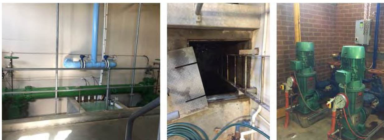
Figure 3-10: Clearwater Inspection Sump (left), CWT entry access point (middle) and Treated Water Pumps (right)
