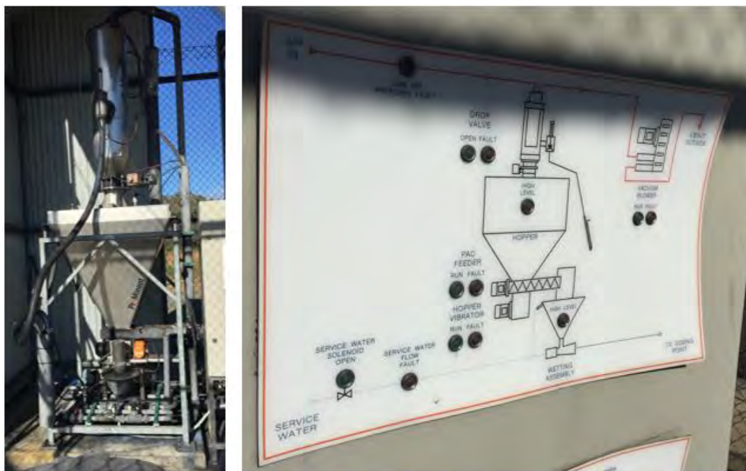
Figure 3-16: PAC Batching and Dosing System
