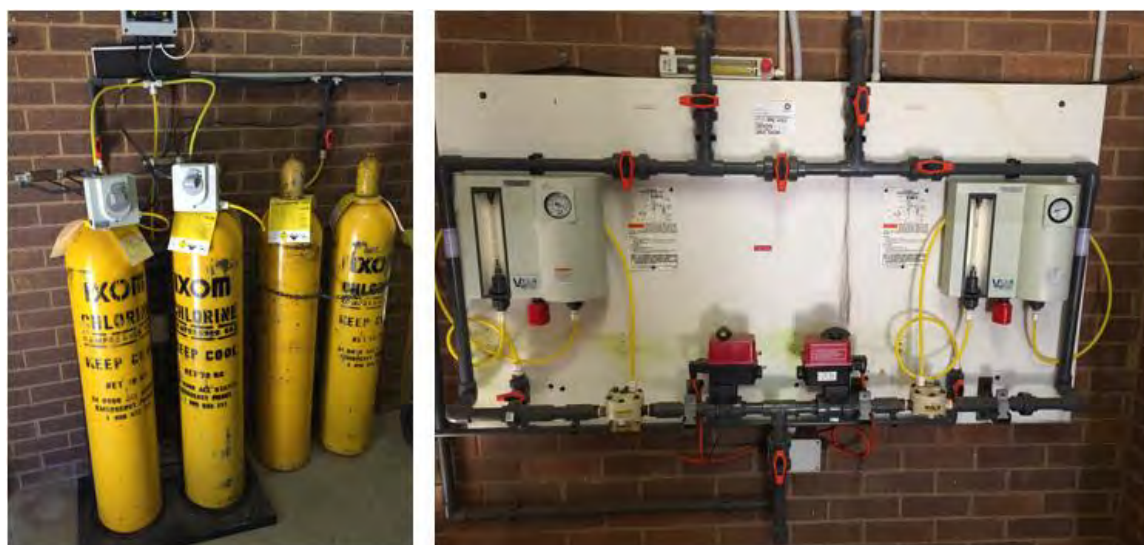
Figure 3-18: Chlorine Gas Dosing System
