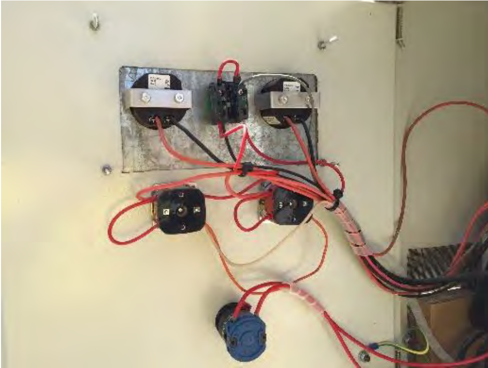
Figure 16-14: Sandy point SPS MCC door wiring
