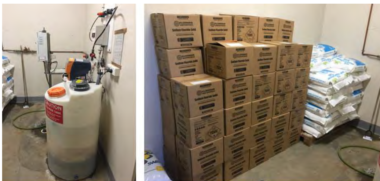
Figure 3-17: ProMinent FluorSat 5-250 and Sodium Fluoride Supply
