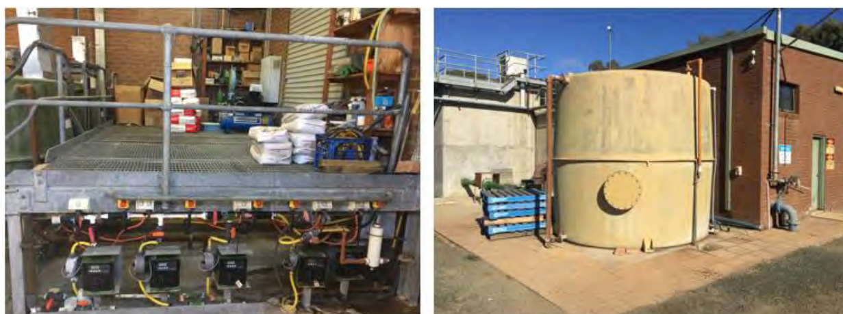
Figure 3-15: Alum (and Soda Ash) Dosing Pumps (left) and Alum Storage Tank (right)
