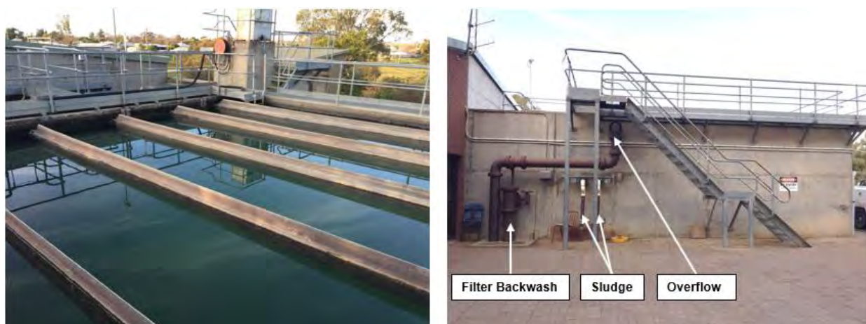
Figure 3-4: Sludge Blanket Clarifier (Pulsator) and Waste Outlet Lines
