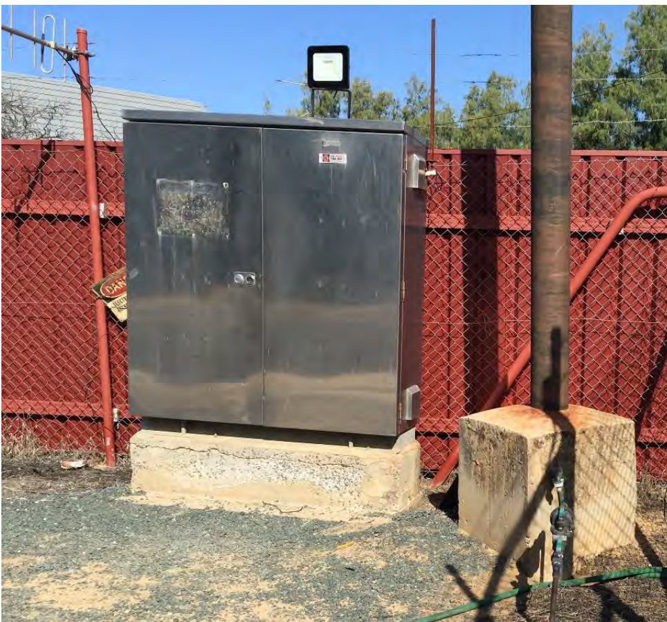
Figure 16-18: Palmer St SPS MCC panel external
