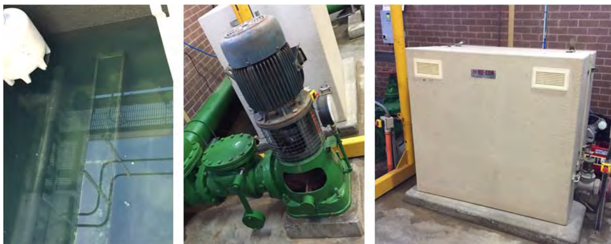
Figure 3-9: Backwash Launder (left), Pump (middle) and Air Scour Blower (right)
