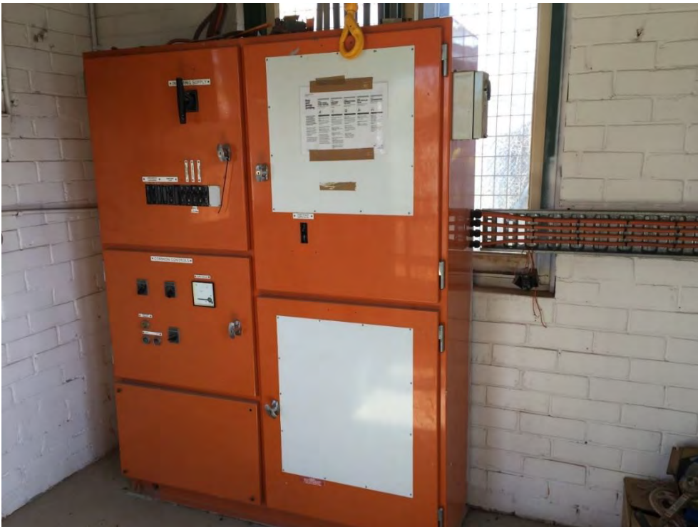
Figure 16-6: Queen St SPS old power MCC panel
