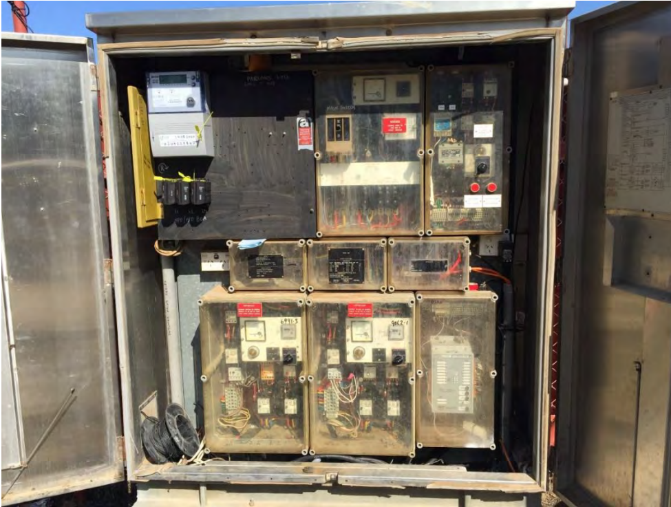
Figure 16-19: Palmer St SPS MCC panel / control panel internal
