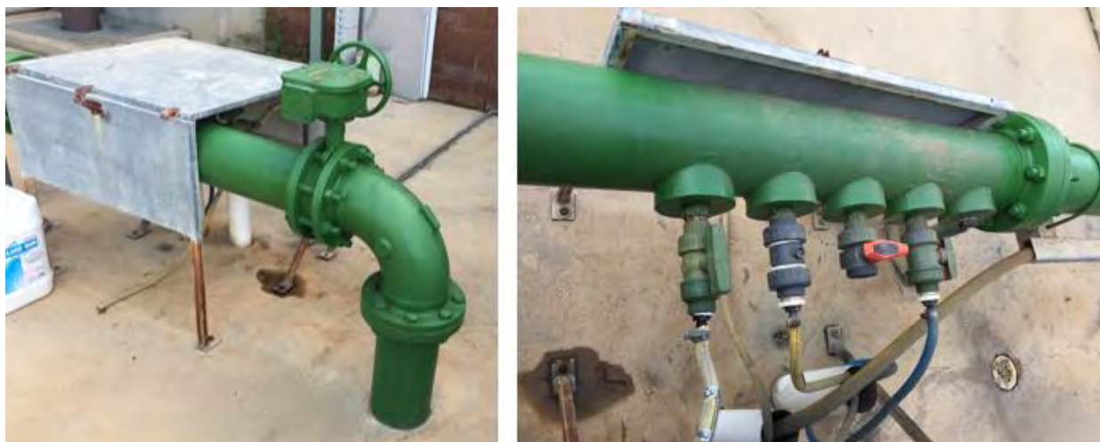
Figure 3-1: Raw Water Inlet and Pre-dosing
