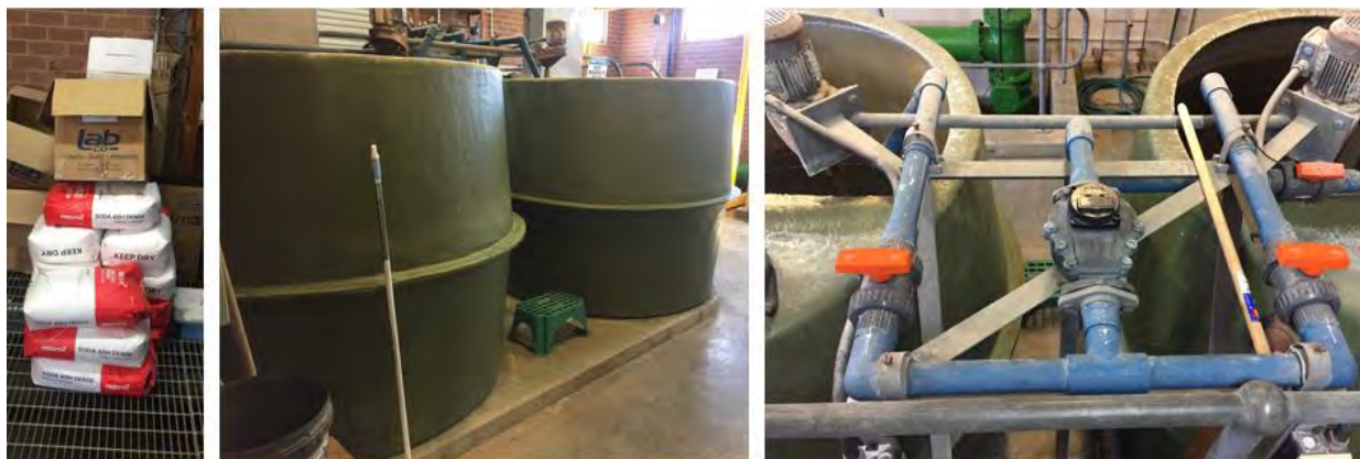
Figure 3-14: Soda Ash Supply and Batching System
