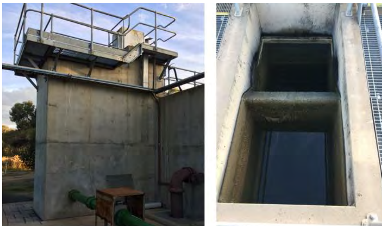
Figure 3-3: Inlet and Vacuum Chambers (left), Inlet Weir (right)
