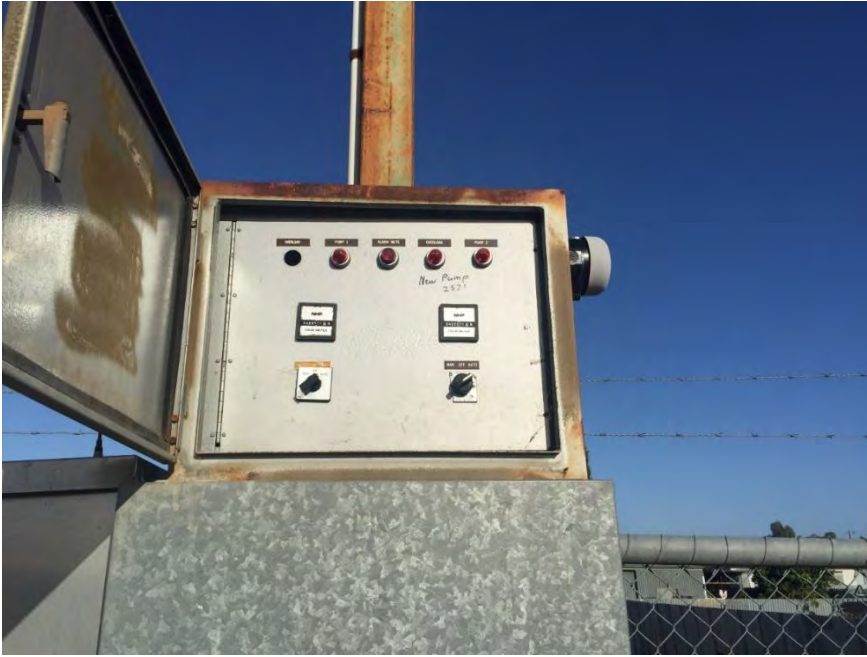
Figure 16-2: Stephen St SPS MCC panel – this panel is to be replaced
