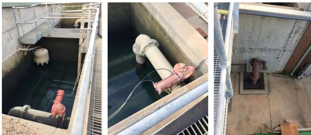
Figure 3-7: Gravity Sand Filters (left), Filter Inlet Pipe (middle) and Backwash Discharge Line (right)
